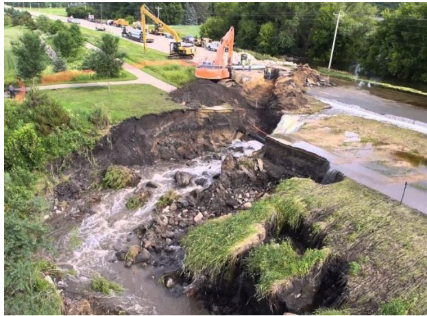
Figure 13. Flood Damage on County Road 16, Shakopee, June 27, 2014 (Noess, 2014)
